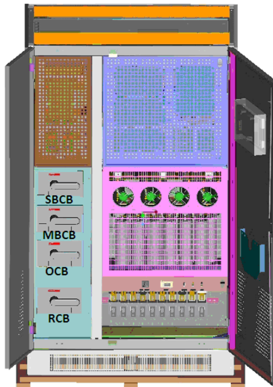
Figure 12: 160 KVA output filter capacitor and disconnecting switch
