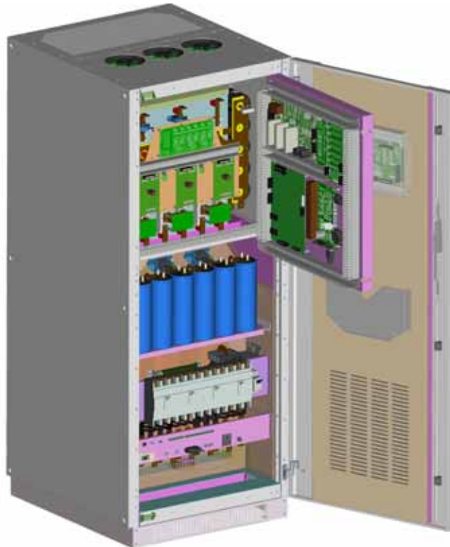
Figure 2-20: 80~120KVA UPS Physical Model of Internal Door
